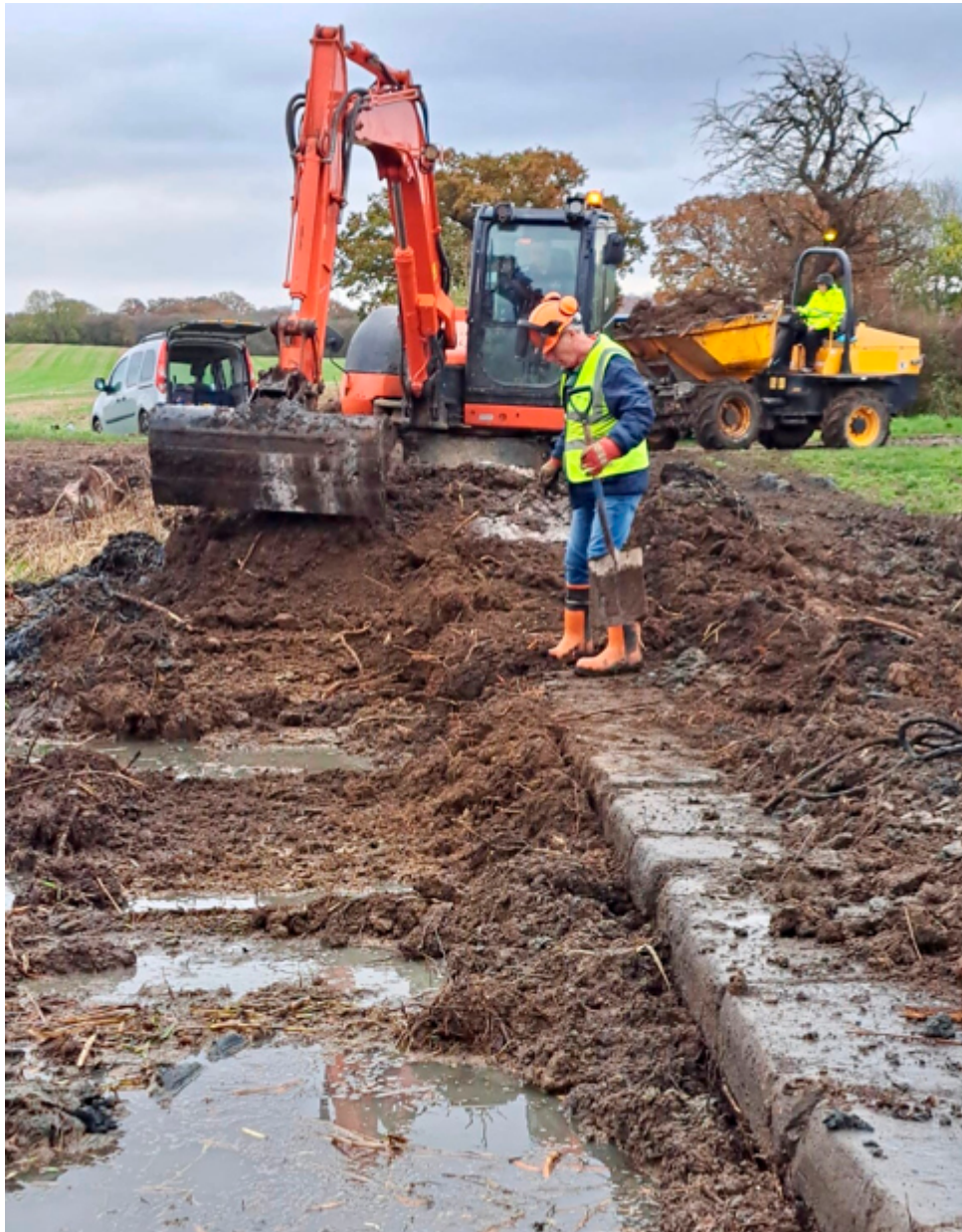
The wharf exposed
