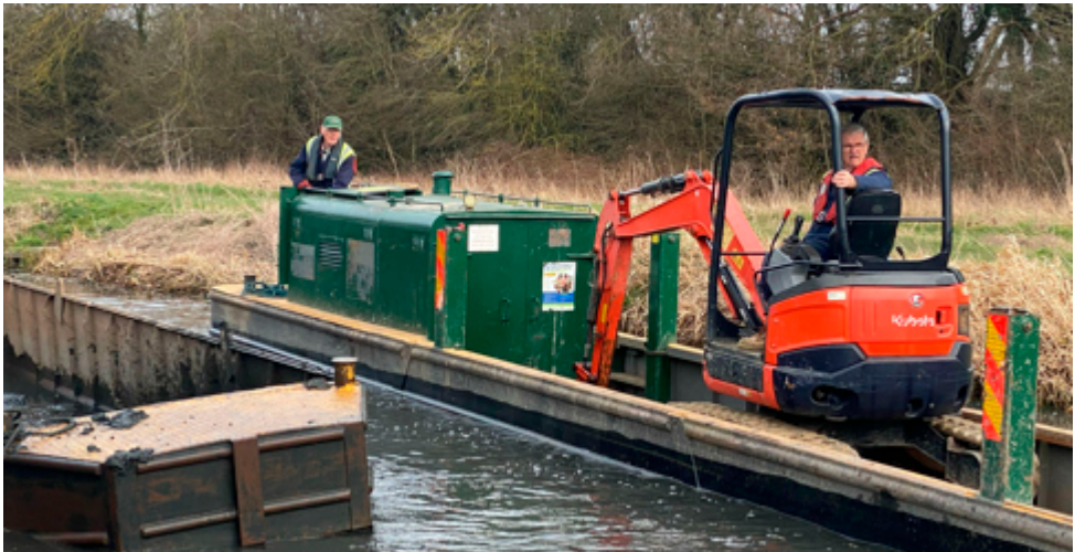
Betty with the on-board excavator during silt removal works.
